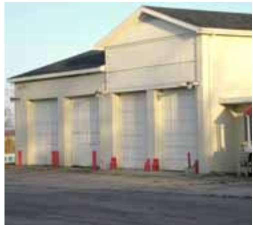
The four-bay auto and repair shop
